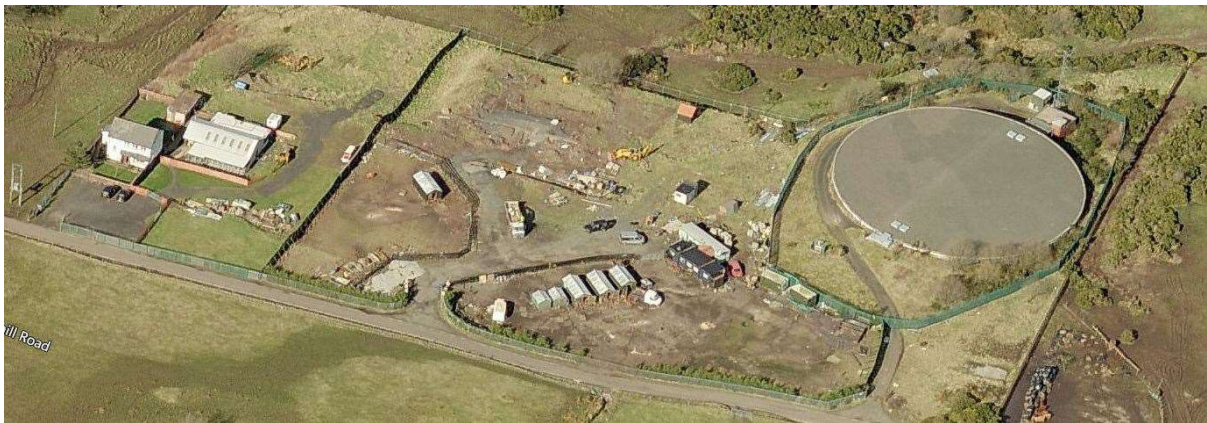
Aerial view during house construction
